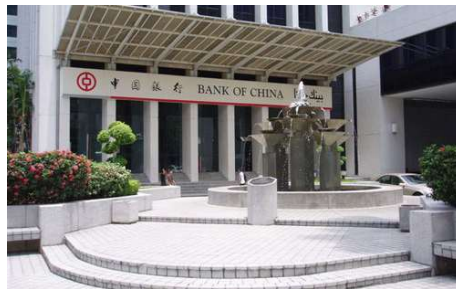
Bank of China, Ampang
