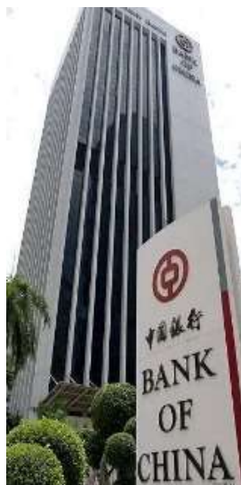
Bank of China, Ampang
